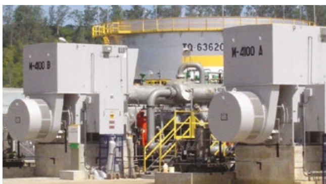
Synchronous motors SEF900 (Ex-p), 3,600 kW, 13,200 V Application: reciprocating compressors (petrochemicals)
